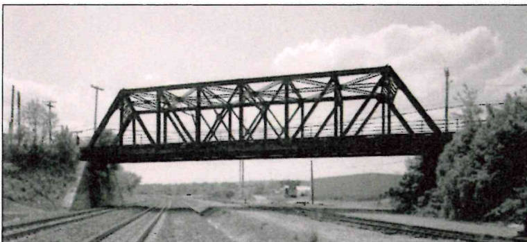
West Street Bridge (1913), Westerly, Rhode Island
